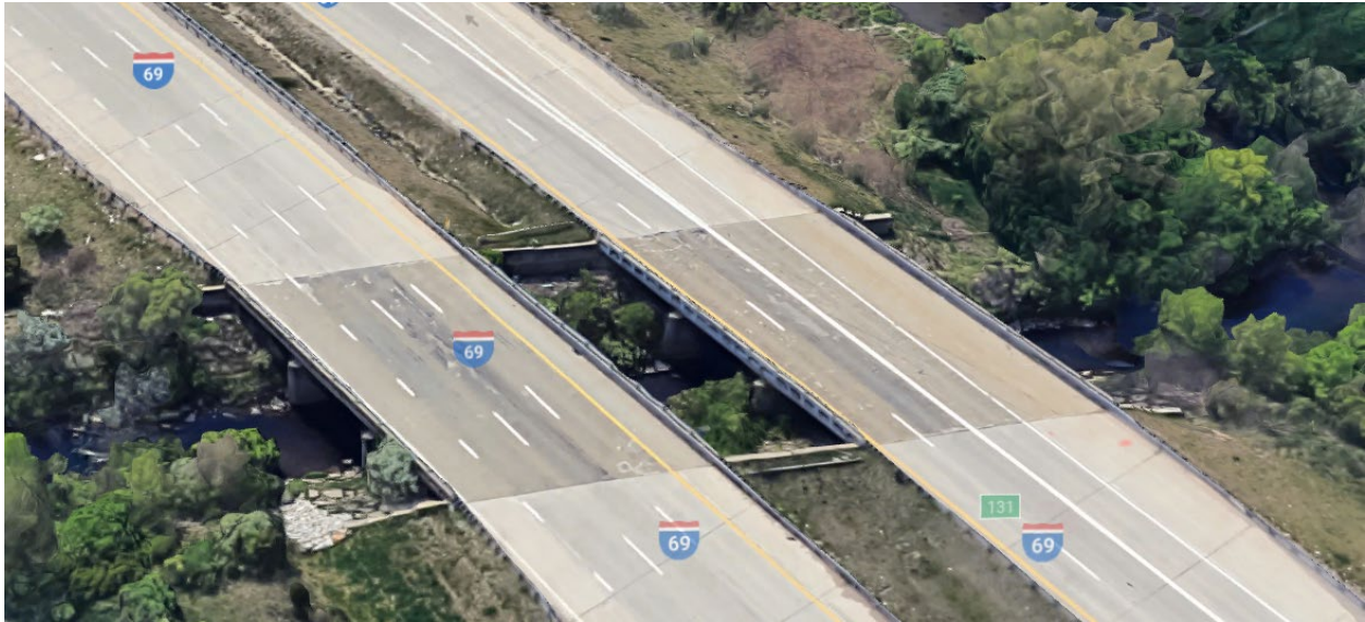
Figure 34. Google Earth 3D Screen Capture of Bridges ID 25125042000B023 and 25125042000B024 along I-69 lxx
