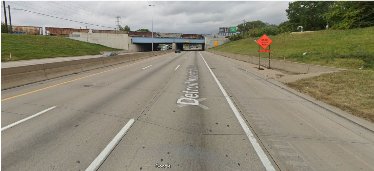
Figure 32. I-94 Google Street View
