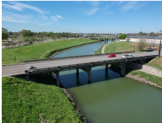
Figure 37. Bridge Deck in Houston, Texas lxiii
