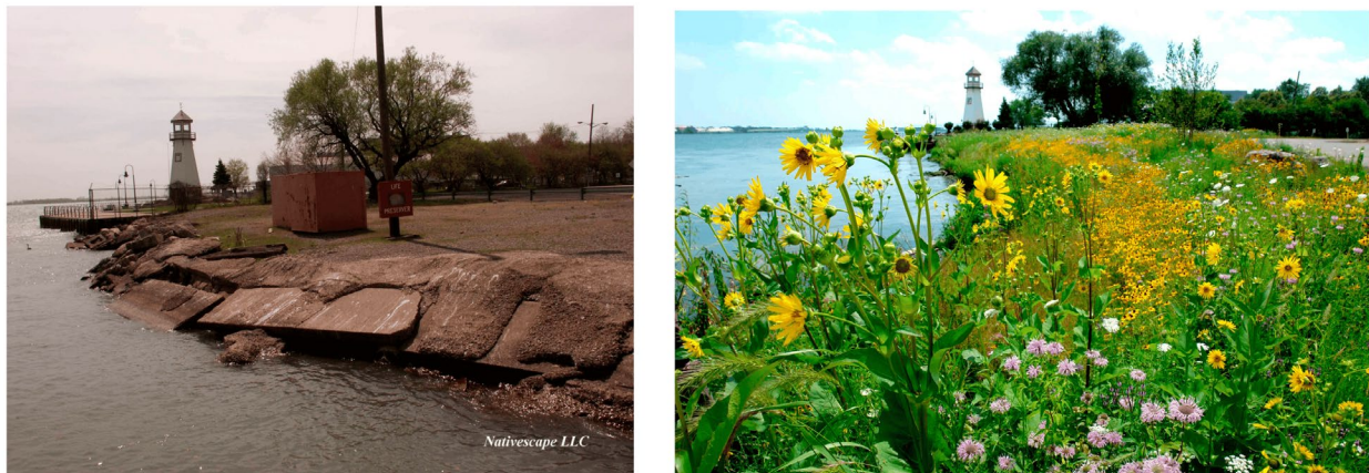
Figure 30. Living Shoreline at Rogue Power Plant, Michigan (Left–Before, Right–After) lxviii
